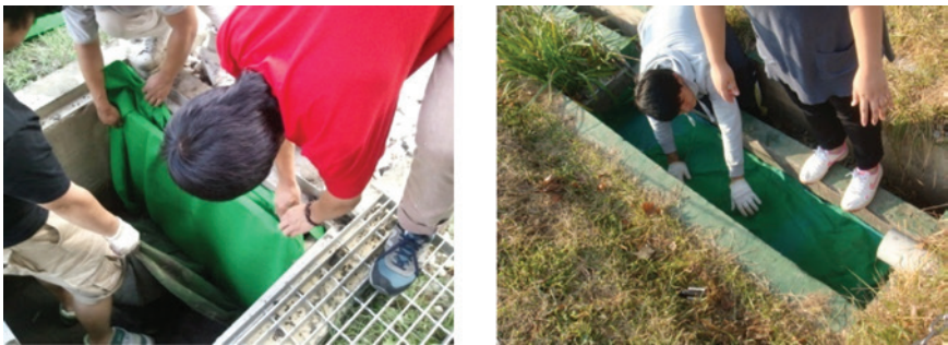
Figure 12.11 As part of the non-routine maintenance, geotextile fabric was replaced in the pretreatment tank of the infiltration trench ( above left ) and hybrid constructed wetland ( above right ).
