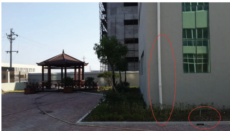
Figure 8.5 Disconnection of roof downspout and rain garden.
