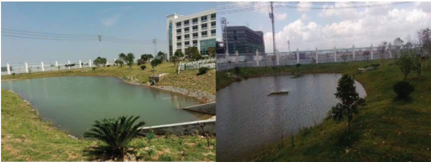
Figure 8.3 Detention ponds in the industrial park. All stormwater from the campus must be discharged to the ponds.
