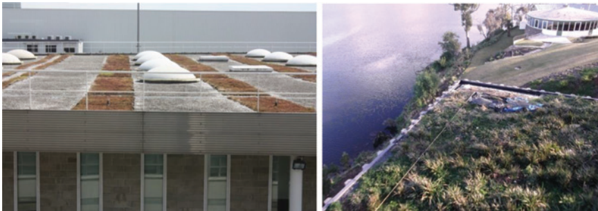
Figure 9.6 Left: Extensive green roof, Charles de Gaul airport. Right: Restoration work on intensive green roof at MONA (Museum of Old and New Art), Hobart, Tasmania.
